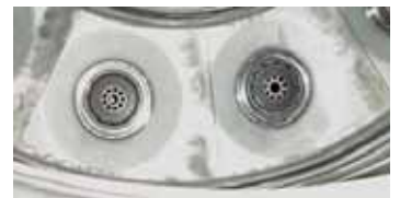
New C50 combustor splash plate repair by brazing
