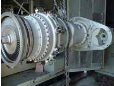
Saturn hoisted out of its package
